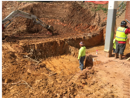
Survey Layout and Footing Excavation
