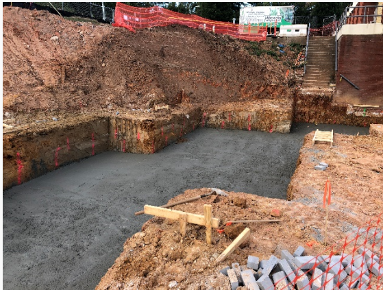
Retaining wall foundation and rebar
